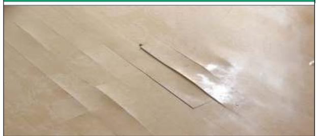
Figure 1. Moisture and pH problems led to strip failure, stressed vinyl composition tile and efflorescence in the seams.
