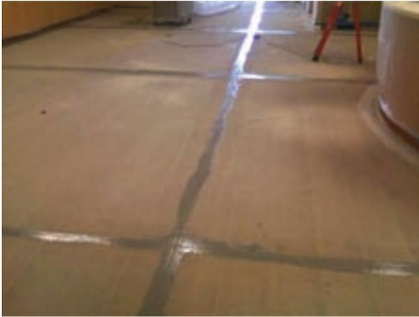
Some of the many aspects of moisture mitigation contractors such as those like Resource Arizona do is using epoxy in the joints and shot blasting the floor to remove the emulsified adhesive and to open the pores in the concrete to prepare it for the next step.
