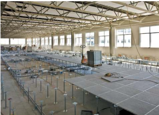
Access flooring under construction.
